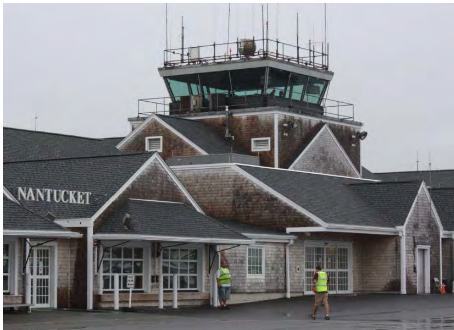
Figure 7-35 Air Traffic Control Tower Rehabilitation – Phase 2 - RECOMMENDED
